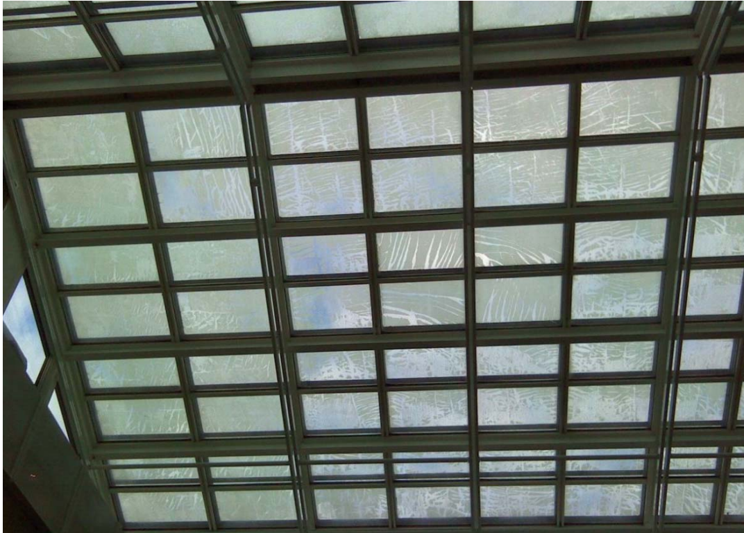
IATA's skylight before renovation
